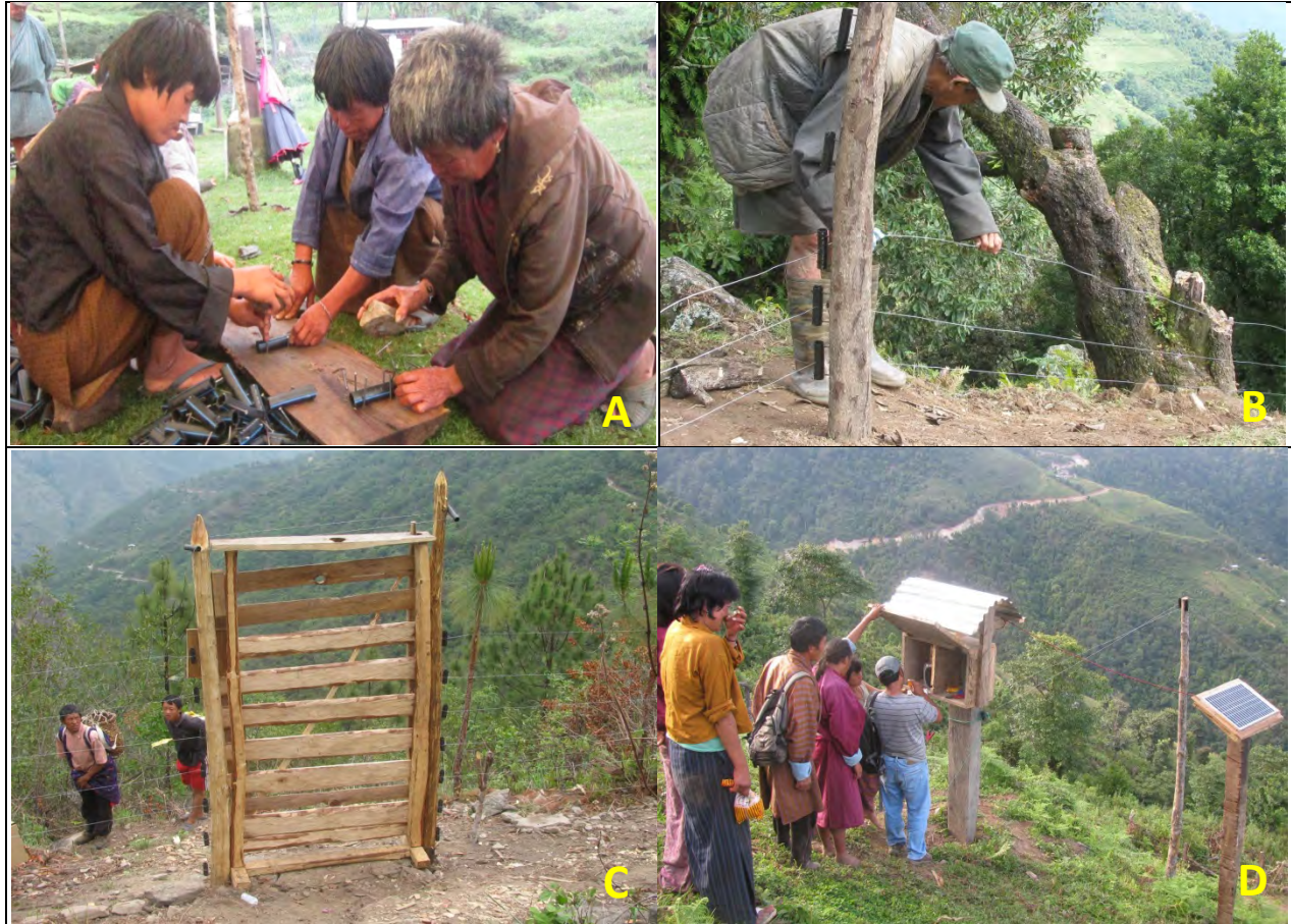
Figure 5. Using readily available materials in FEF: Elderly women fabricating electric fence insulators using HDPE pipe and iron nails (A). Elderly man fixing GI wire and HDPE insulators to the wooden post (B); Entry/Exit gate constructed from local materials (C); Locally made wooden box to contain energizers, batteries and other accessories (D)
